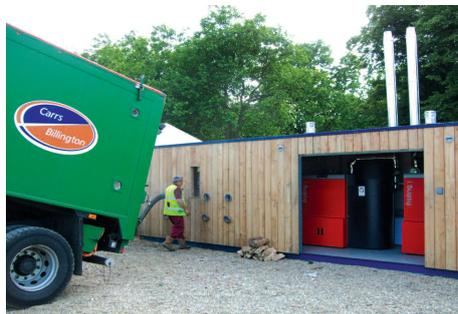
**3** Get the fuel store as close to the boiler as possible. By cutting down auger/transfer distances to a minimum, you lessen fuel jamming issues and further fuel degradation.
