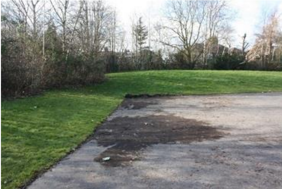
Figure 2 – Silt Deposit from Run Off on Sports Pitch next to Grass Embankment
