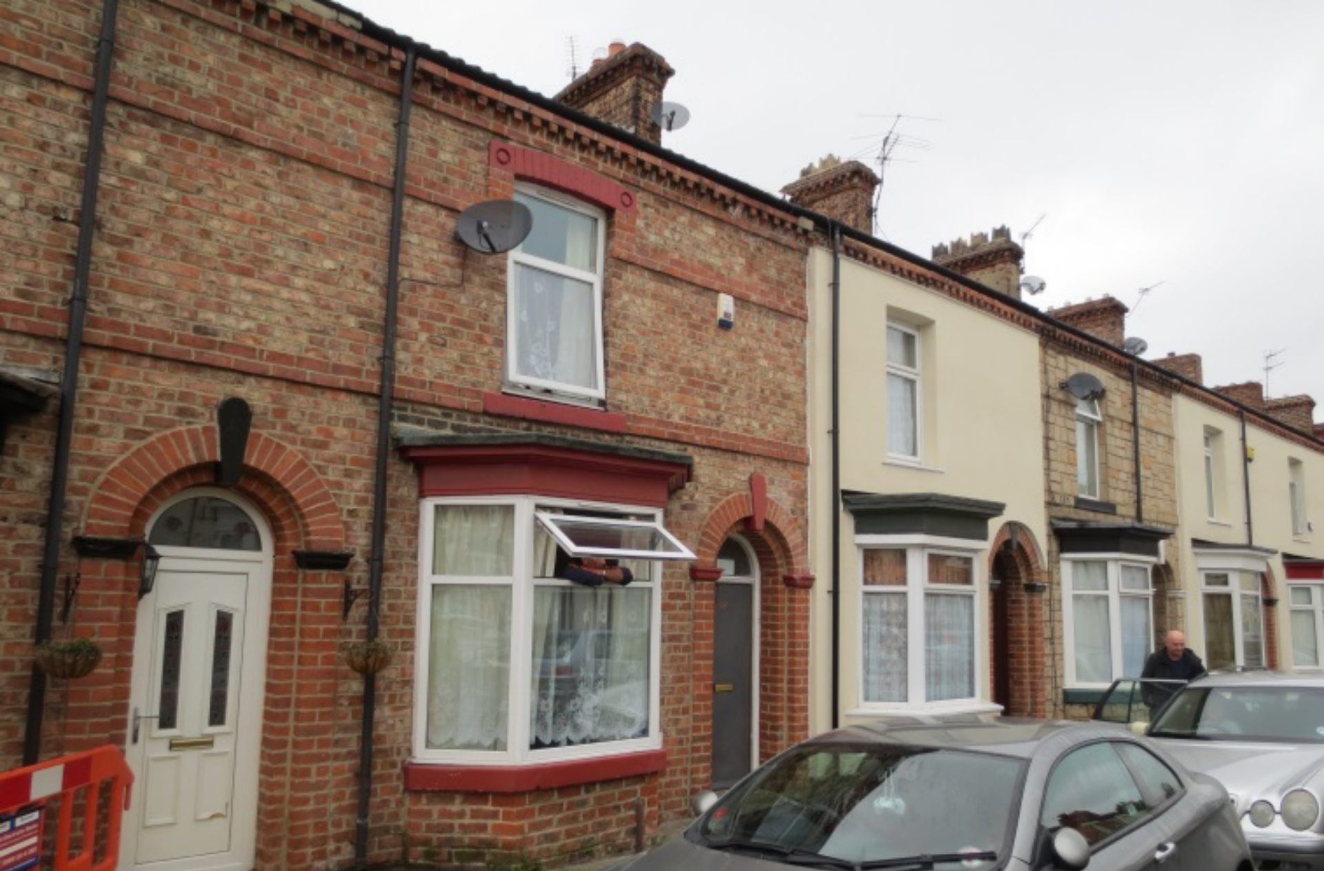
■ Partial treatment of terraces
