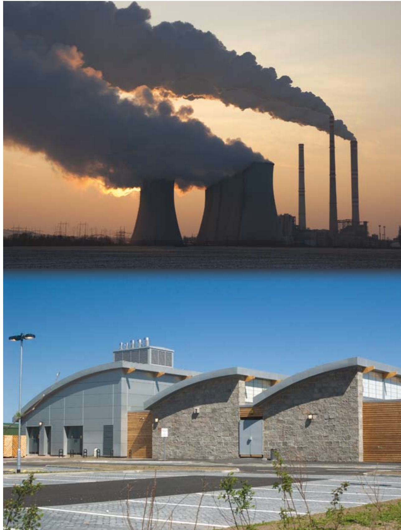
Figure 2: Centralised power generation wastes approximately 60% of primary energy in the form of heat rejected into the atmosphere. Decentralised generation captures this heat and is 80-90% efficient
