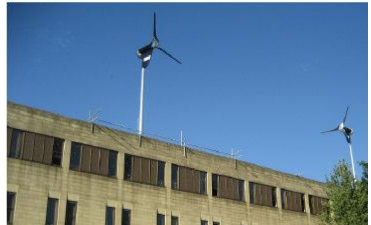
Proven 6kW turbine, Kirklees Civic Centre
